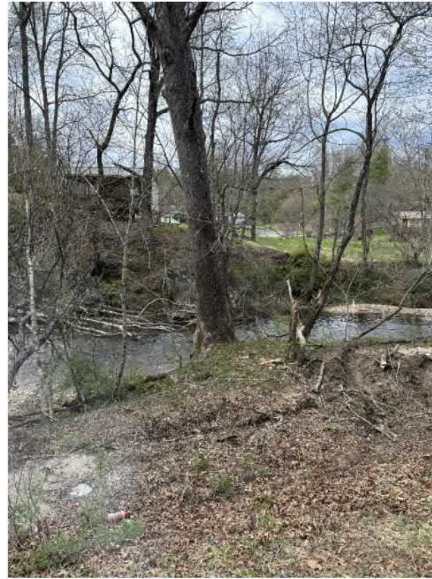
NORTH APPROACH AT END BENT NO. 2 LOOKING SOUTH
