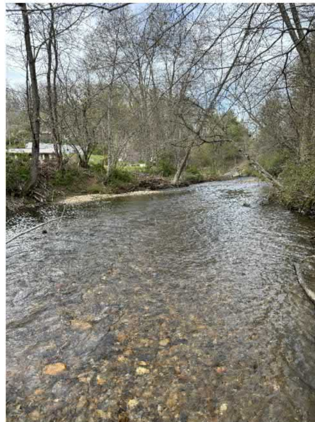
SOUTH APPROACH AT END BENT NO. 1 LOOKING NORTH
