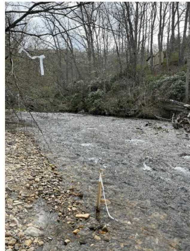
INTERIOR BENT NO. 1 LOOKING SOUTHWEST UPSTREAM
